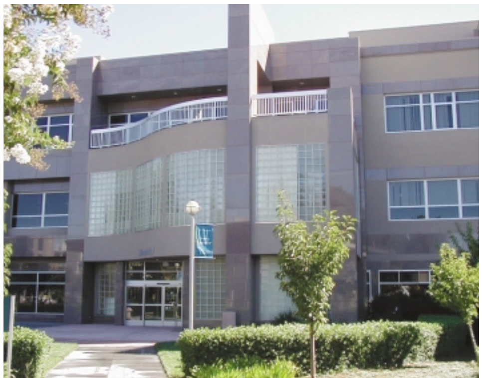
Kaiser's Walnut Creek, California, hospital campus.
